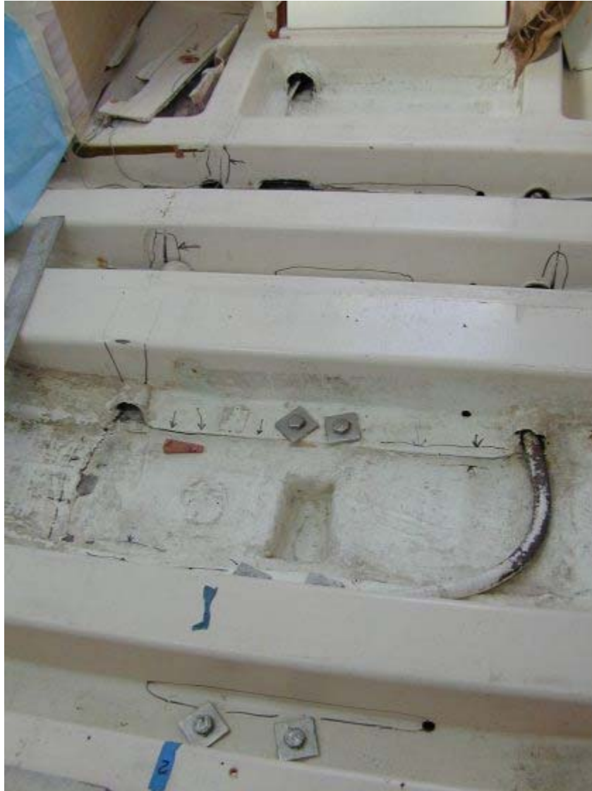
Grounding damage. Note cracks near limber holes and wire runs. Floor bond to hull failed in some areas.
